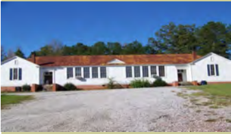
Woodworking Education Center 10544 Hwy 17, Maylene, AL 35114
